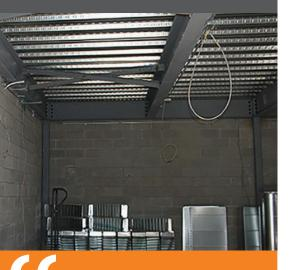
The many design alterations throughout the construction made the use of BlazeMaster CPVC a more easily adaptable system than steel, which would have required refabbing in the field.
