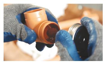
Apply a heavy, even coat of cement to the outside of the pipe end, then a medium coat to the inside of the fitting socket. Pipe sizes greater than 2 inches (50mm) should receive a second coat of cement on the pipe end. Don't allow the solvent cement to puddle within the fittings and pipe.
