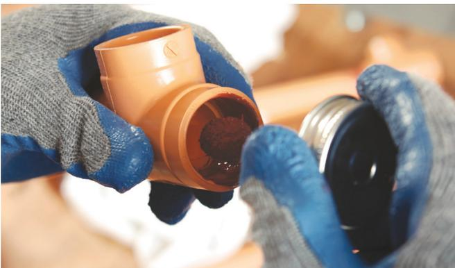
Apply a heavy, even coat of cement to the outside of the pipe end, then a medium coat to the inside of the fitting socket. Pipe sizes greater than 2 inches (50mm) should receive a second coat of cement on the pipe end. Don't allow the solvent cement to puddle within the fittings and pipe.
