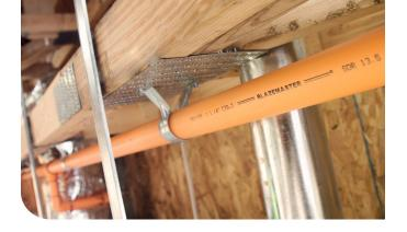
This approach enabled Alwest to use only one expansion loop to address expansion and contraction. Expansion loops are U-shaped configurations placed in the middle of a run of pipe that allow pipe to move back and forth. Custom calculations of expansion loops, offsets and changes of directions can be found here.
