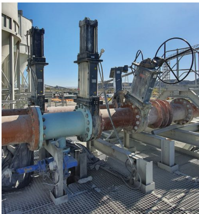
Weir's DELTA INDUSTRIAL knife-gate valves in a tailings application at a gold mine.
