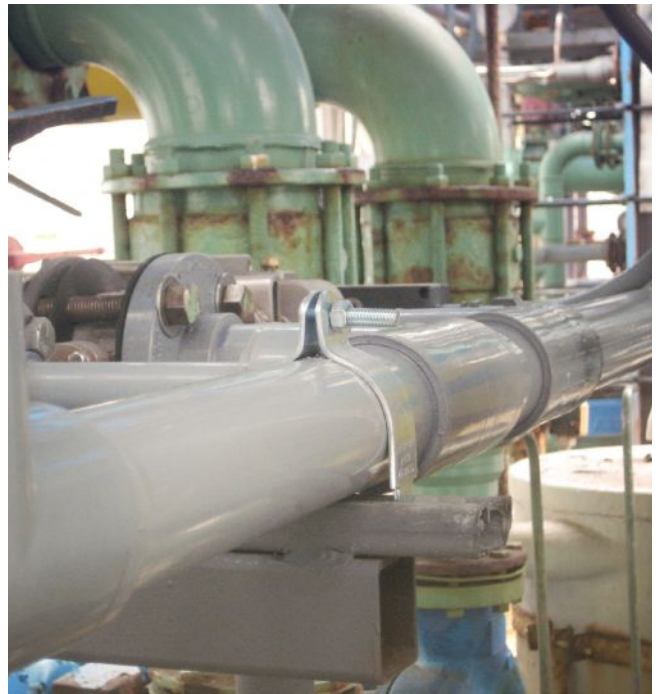
Corzan CPVC pipes offer an alternative to steel pipes in mineral processing operations. Photos: The Lubrizol Corporation
