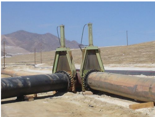
In a tailings system, spigot pipes tee off the main tailing distribution line to feed various sections of the containment area. Each spigot features an isolation valve to control the flow of tailings to a specific zone, ensuring the material is uniformly distributed across the containment surface. Photo: Emerson
